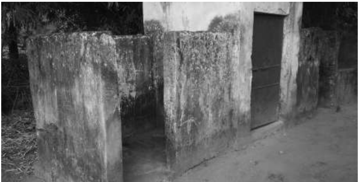
21020101801 – MANGLUPADA PS, TALMAL AREA, JHARSUGUDA, Existing Toilet Status as on 15.01.2015
